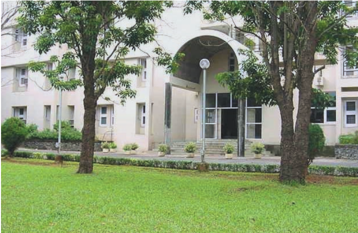
Front View of the Guest House
